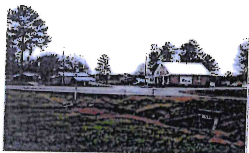
Figure 50. Villanow Community, Walker County Georgia
