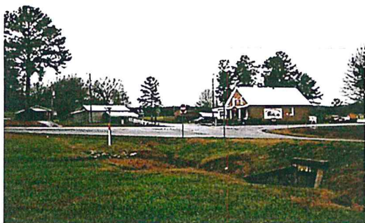
Figure 50. Villanow Community, Walker County Georgia
