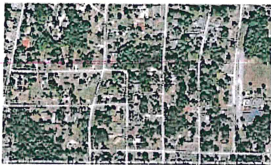
Figure 50. Residential development in the Mountain View area
