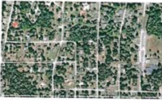
Figure 50. Residential development in the Mountain View area
